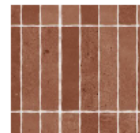
Faux stone facade (entry structure)
